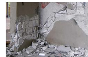
Dazio et al. (2009b), L'Aquila earthquake Web diagonal tension, flange buckling and crushing
