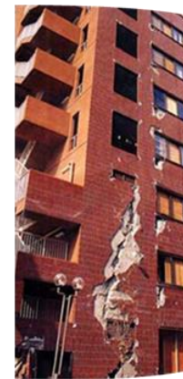
Maffei and Yuen 2007 Kobe earthquake, Diagonal Tension
