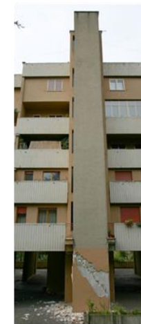
Dazio et al. (2009b), L'Aquila earthquake Web diagonal tension, flange buckling and crushing
